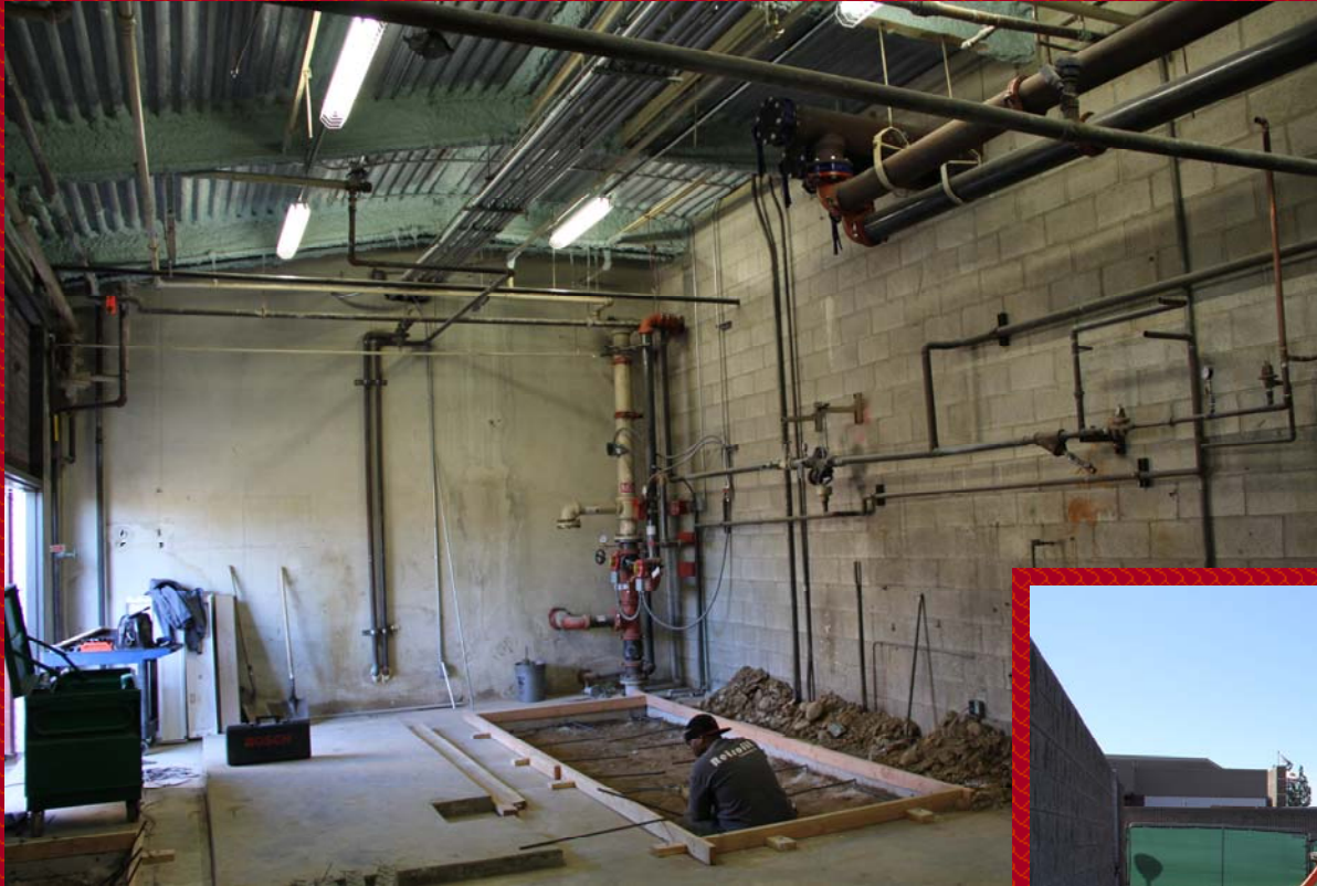
Chiller Replacement Project
